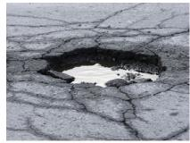
is asphalt material, usually from an asphalt plant, that is installed in the pothole area. Usually the damaged material is removed and the hot mix is placed at a sufficient depth and compacted. This is usually a better long-term option. Typically, communities use cold mix material to patch roads. This is usually a short-term fix but is cheaper than the alternative hot mix.
