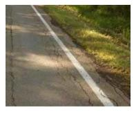
Wheel track and edge cracking is cracking that occurs on the edge of the asphalt or within the typical wheel tracks. These types of cracks usually run parallel to the outer edge of the pavement and cracking is increased by continuous traffic loading. Edge cracking can be caused by weakened base or subgrade near the edge of the pavement. This type of cracking can lead to raveling, which means that the edge has broken off from the main asphalt road.
